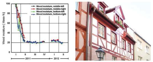
Fig. 6. Course of the wood moisture (left) and view of the building after restoration (right).
